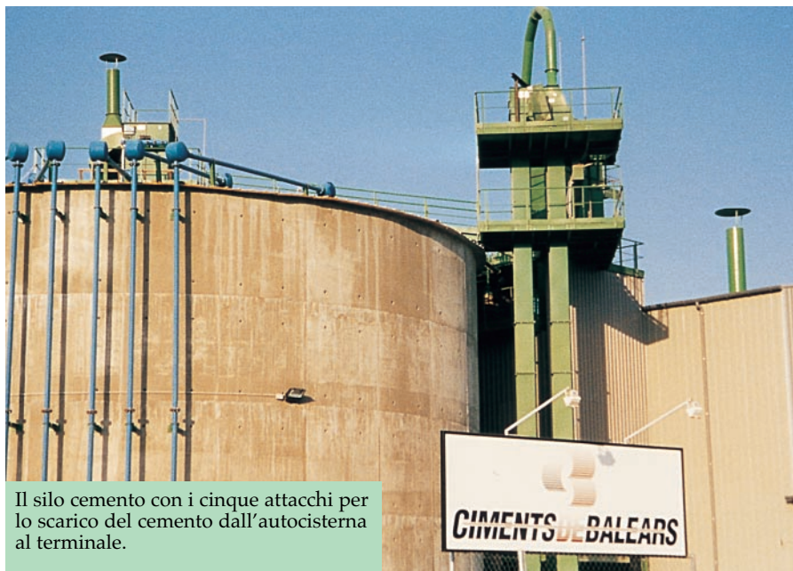
The cement silo with the five connections for unloading the cement from the tanker-truck at the terminal.
